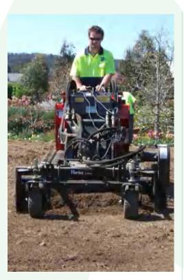
Preparation and cultivation of the site subgrade is important to be carried out prior to installation of final topsoil.
